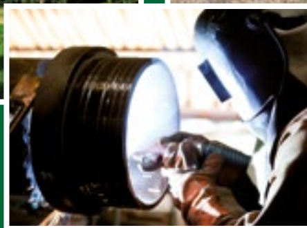
Welding of the spigot end and pipe
