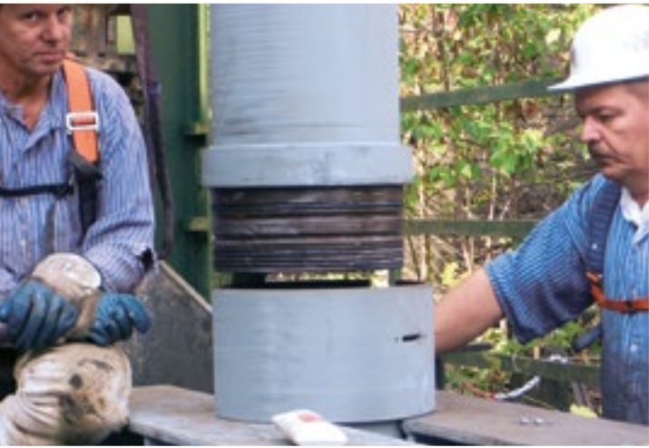
Installation of a ZSM Pipeline
